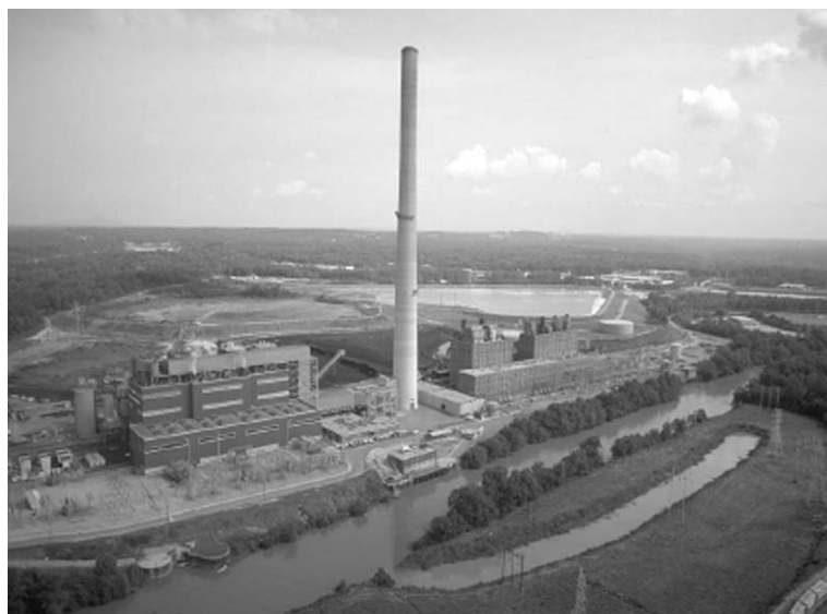
Georgia Power's Plant McDonough in Atlanta
