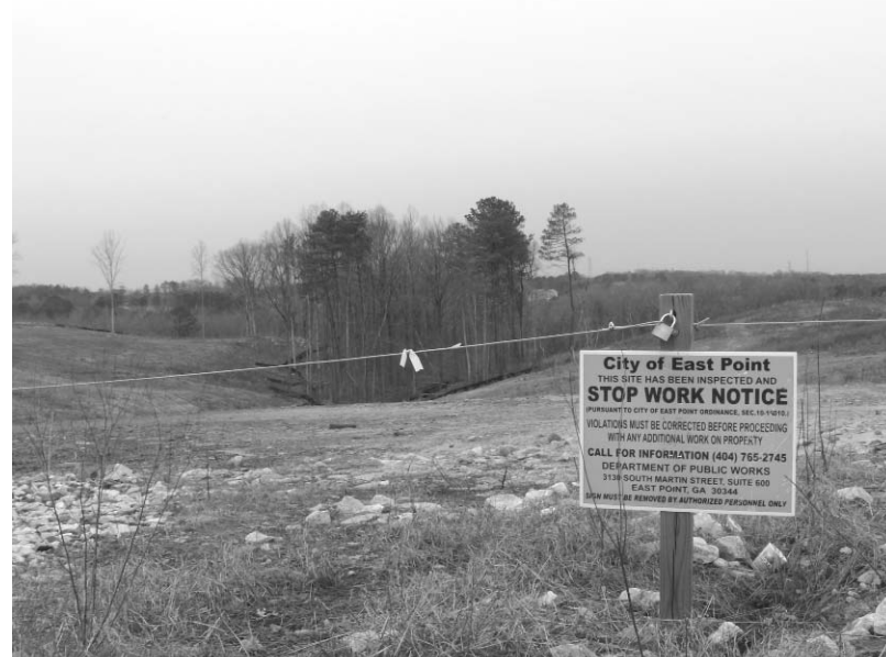
Under a stop-work order for more than 2 1/2 years, this residential development in East Point is still not properly stabilized.
