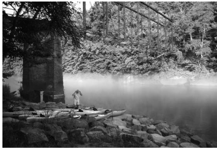
Morning mist at Settles Bridge in Gwinnett County.
