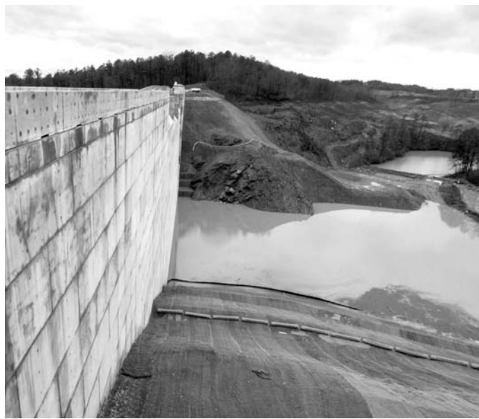
The new Hickory Log Creek Reservoir, which dams a tributary to the Etowah River in Canton, will cost more than $100 million.
