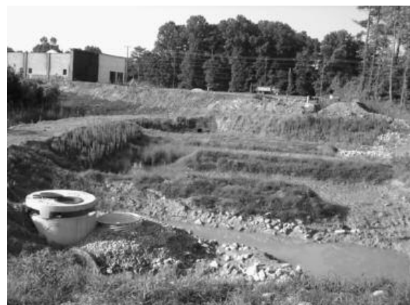
This stormwater detention pond drains to constructed wetlands at the Silverbrooke development in Powder Springs.
